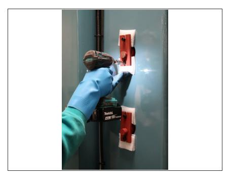
Using a <u>6 MM Hex Socket</u>, center screw the counterweight support brackets into the column, and make sure that the counterweight support is held tightly.
